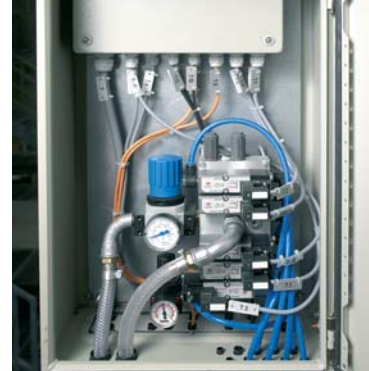
Advanced control technique. ISO-base plate valves. Compact, protected.
