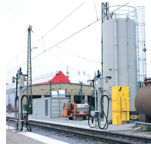
Sand storage silo with filter. Free dust is separated, no exhaust escapes into the working area.
