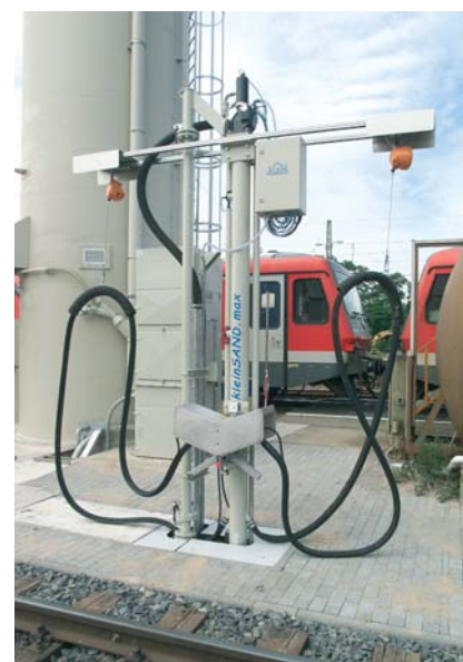
Gravity balancers relieve the weight of the filling valves and retract the hoses into a parking position after use.
